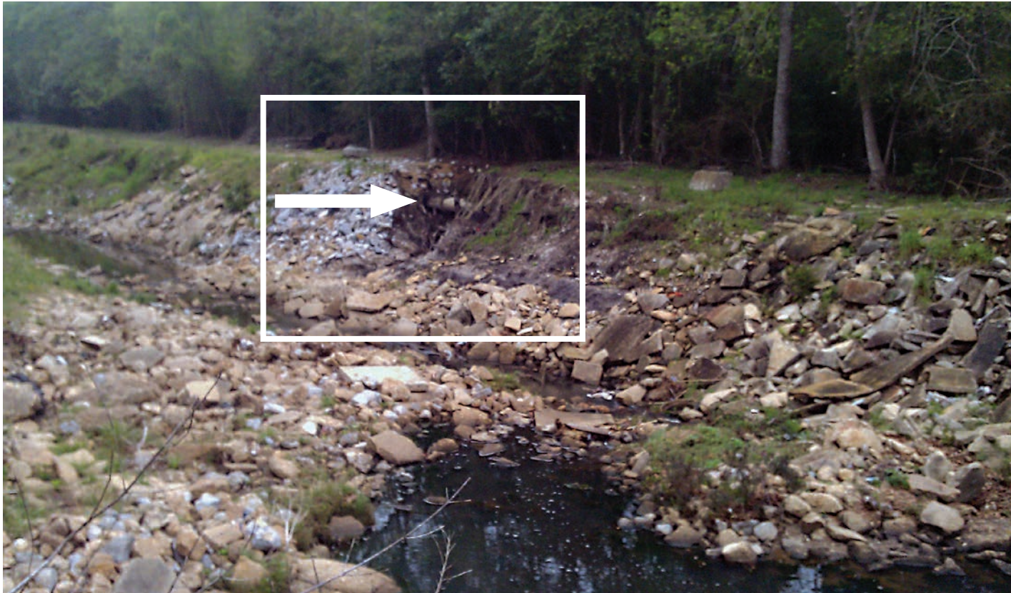
Erosion caused by stormwater runoff threatens infrastructure throughout the watershed. In this photo, bank erosion has exposed a section of sanitary sewer pipe along Twelve Mile Creek, increasing the risk of illicit discharges to the stream.
