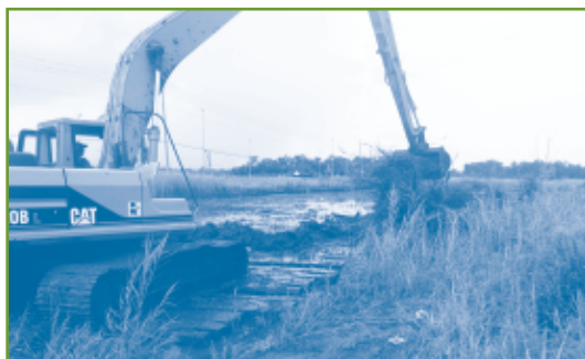
Mitch Dickens of Esfeller Construction operates the long stick excavator at Helen Wood Park
