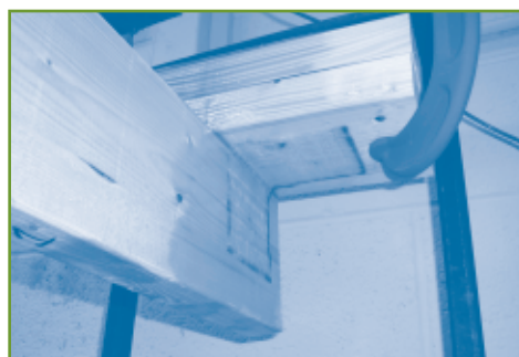
Fiber reinforced polymer connection used to strengthen structures in hurricane vulnerable coastal areas.
