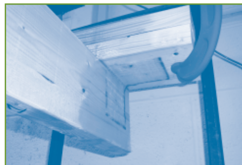
Fiber reinforced polymer connection used to strengthen structures in hurricane vulnerable coastal areas.
