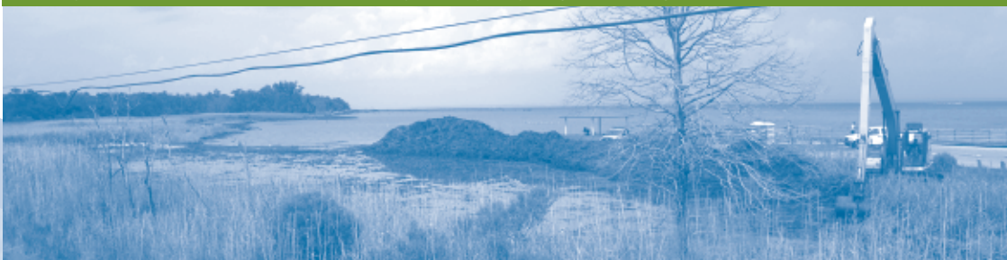
View of the Helen Wood Park marsh excavation from the foot of Dog River Bridge.
