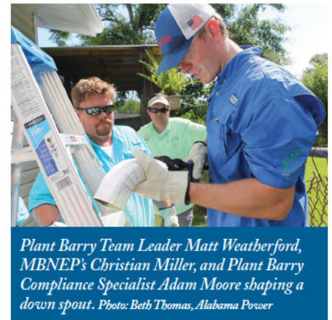
Plant Barry Materialman Terry Coleman assists by capping a gutter. Photo: Beth Thomas, Alabama Power
