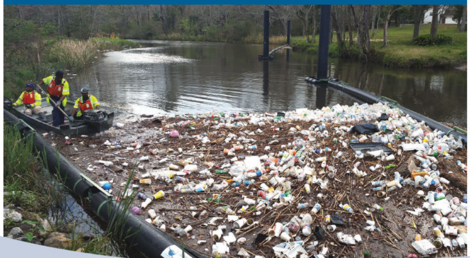
City of Mobile employees removing captured floatable trash from the Bandalong™ Litter Trap in the Eslava Creek Tributary to Dog River. Photo: David Ludwig, City of Mobile
