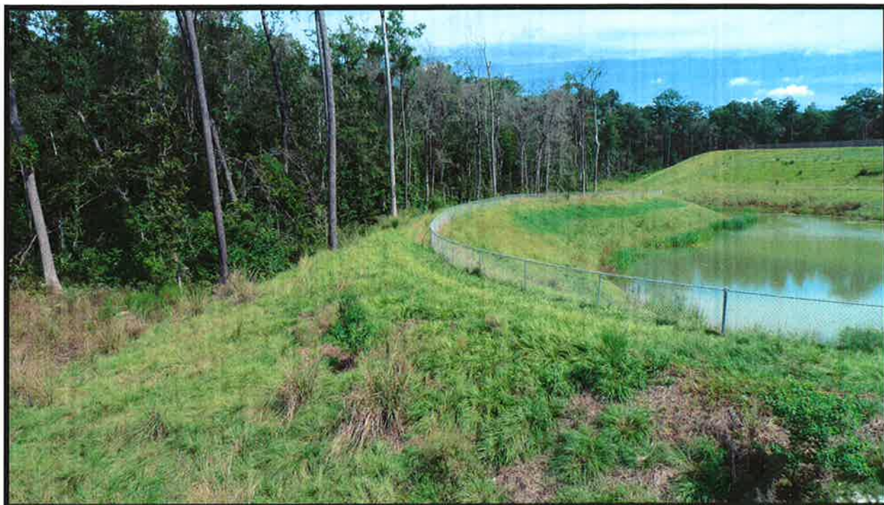
PHOTO 7: Site J2W looking north. Note the re-contouring of the upland buffer to the edge of the wetland line.
