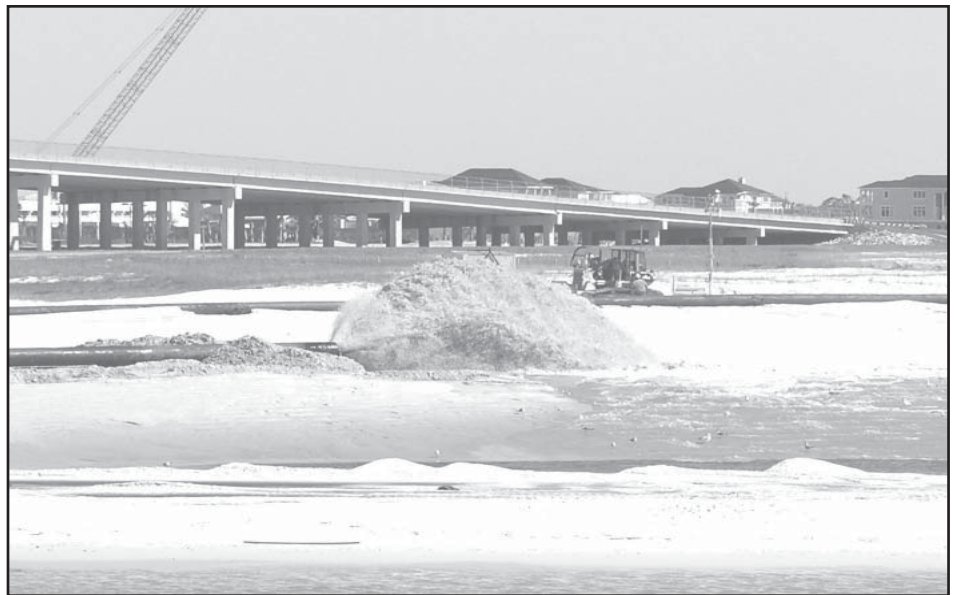
Restoration of Perdido Pass after Hurricane Ivan, Orange Beach, Alabama
