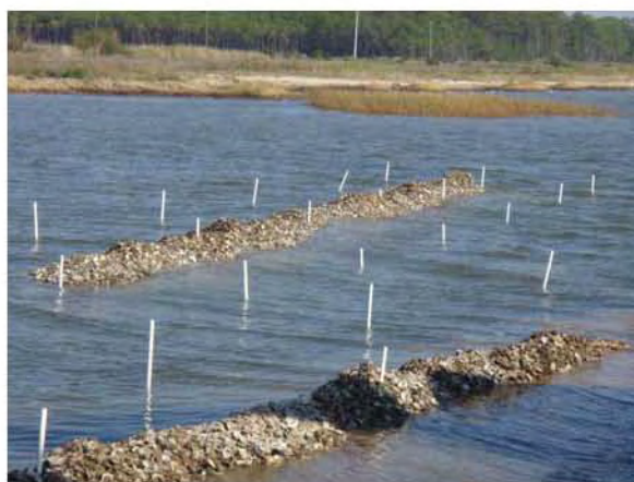
Figure 1: Photograph of one of the breakwater reef complex constructed near Bayfront Park, AL.
