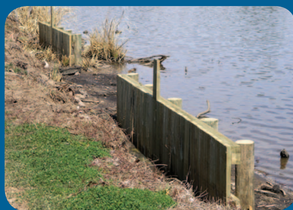
Seven twenty-foot, pile-supported, timber structures were installed along the Dog River Park shoreline with clean sand fill placed behind them to create artificial headlands.
