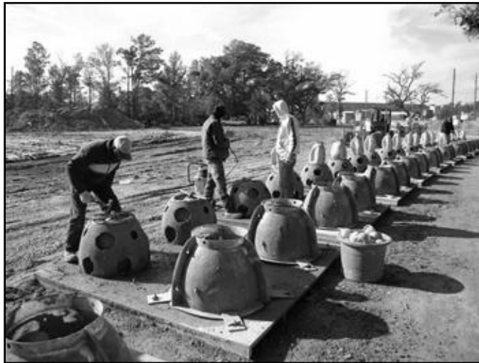
Figure A2: Construction of Reef Balls to be placed along Alabama shorelines under the American Recovery and Reinvestment Act (Photo Courtesy: Jeff DeQuattro/The Nature Conservancy).
