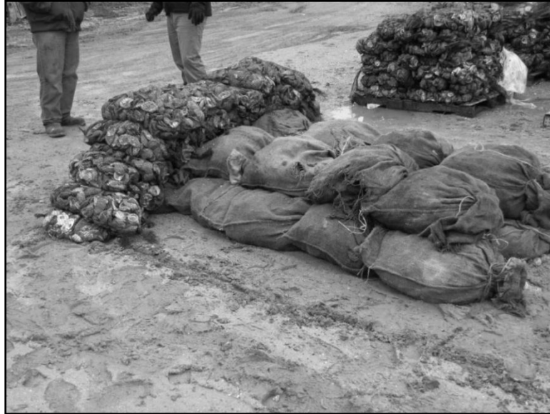
Figure A3: Composition of a bagged oyster shell breakwater to be used at Helen Wood Park, Alabama.
