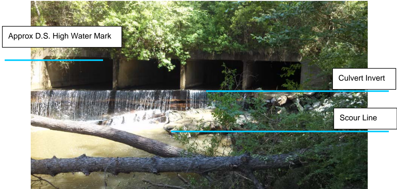
Figure 3-29 Downstream Scour I-10 Culvert – April 29-30, 2014
