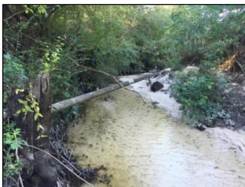
Picture 8: Exposed pipeline in an unnamed tributary to Bon Secour River
