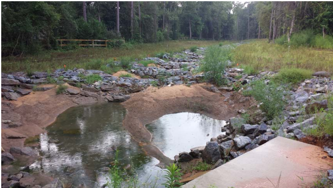
Figure 4.—Sediment deposition in step pool conveyance system cells as a result of land disturbance upstream from site JB1.
