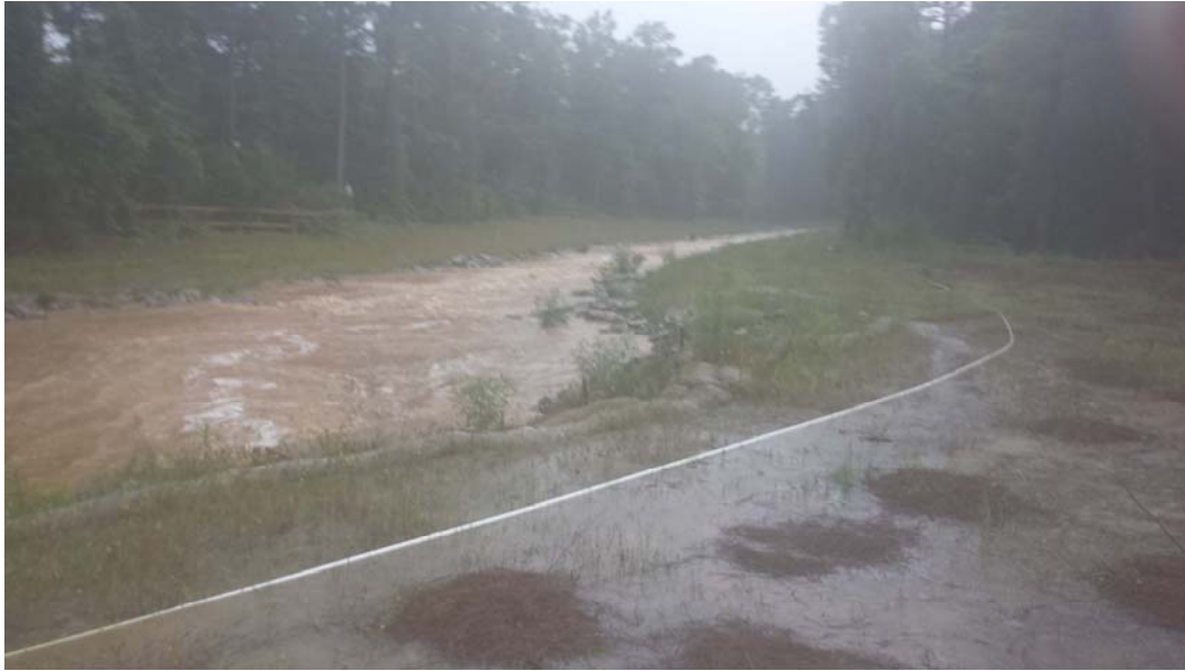
Figure 11.—The step pool conveyance system after an intense storm event with discharge of about 43 cfs on July 11, 2013.
