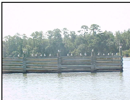
Slotted wave attenuator at entrance of marina
