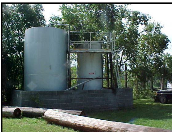
Barriers in place around liquid storage area
