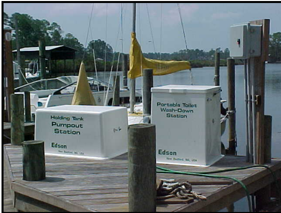
Vessel Pump Out Station
