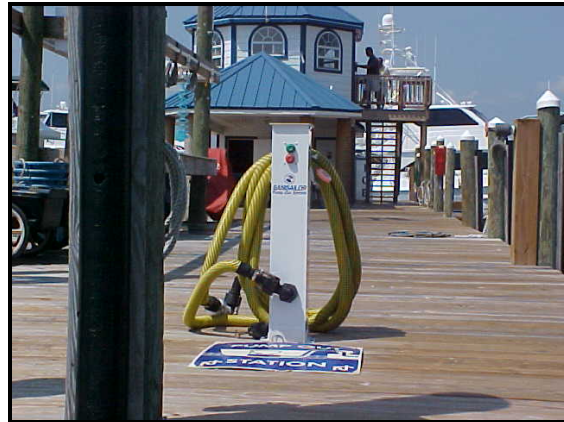
Dockside Vessel Pump Out Station
