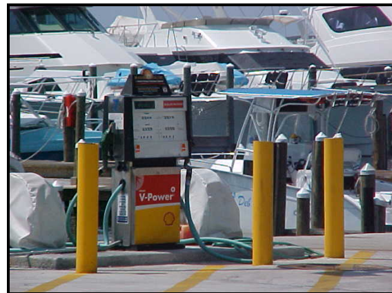
Station location so that spills can be limited to a contained area
