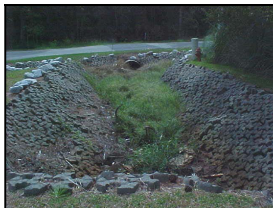
Onsite Infiltration Trench
