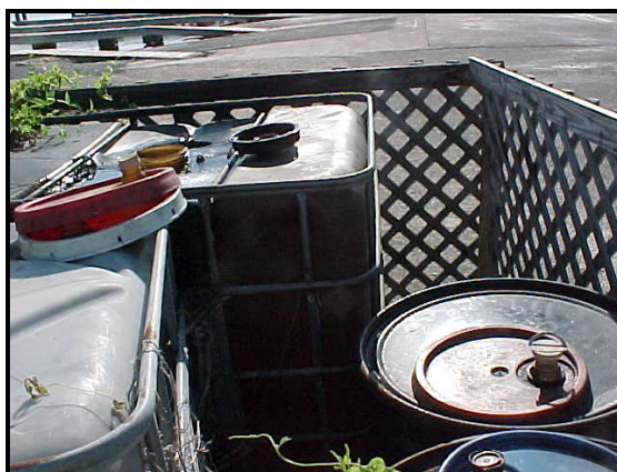
Needs labeling & signage for disposal of liquid waste
