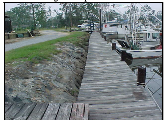
Interesting shoreline stabilization techniques with the use of roof shingles.
