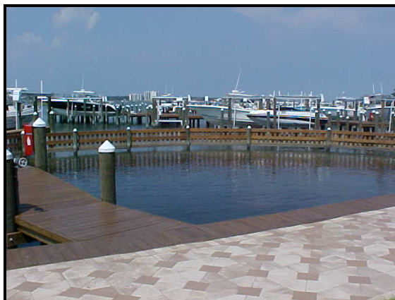
Slotted wave attenuator as protection for SAVs
