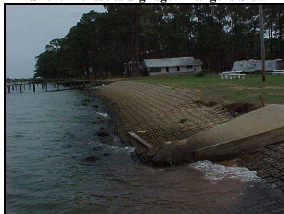
Example of Erosion Due to Wave Energy
