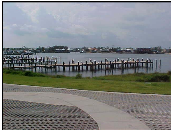
Porous parking and grassed buffer
