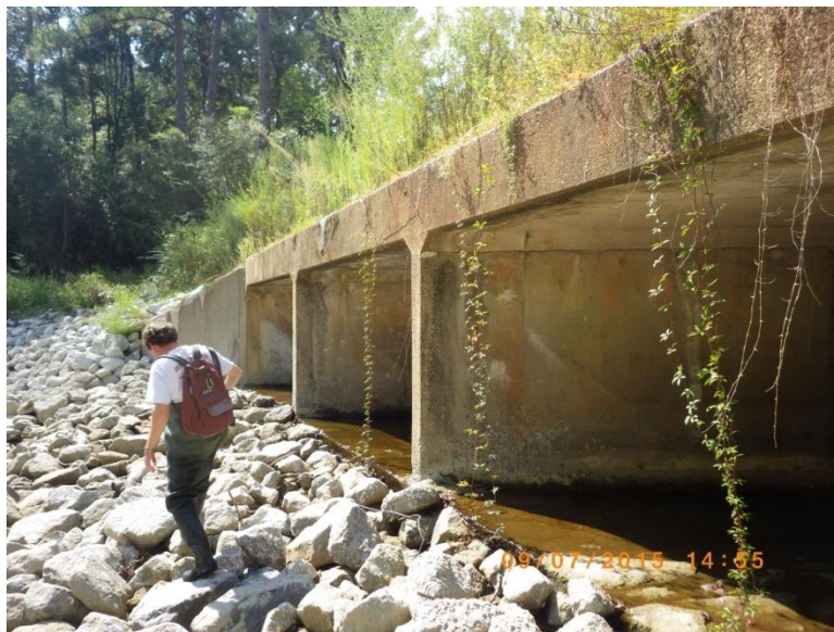
Figure 34: An example of the culvert and rip rap upstream from T0C in September 2015.
