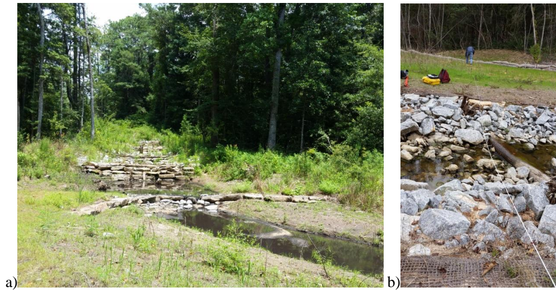
Figure 3: Examples of hard stabilization techniques used in the study area at a) Joe's Branch step pool conveyance (completed 2013) and b) JB1R (completed 2015).
