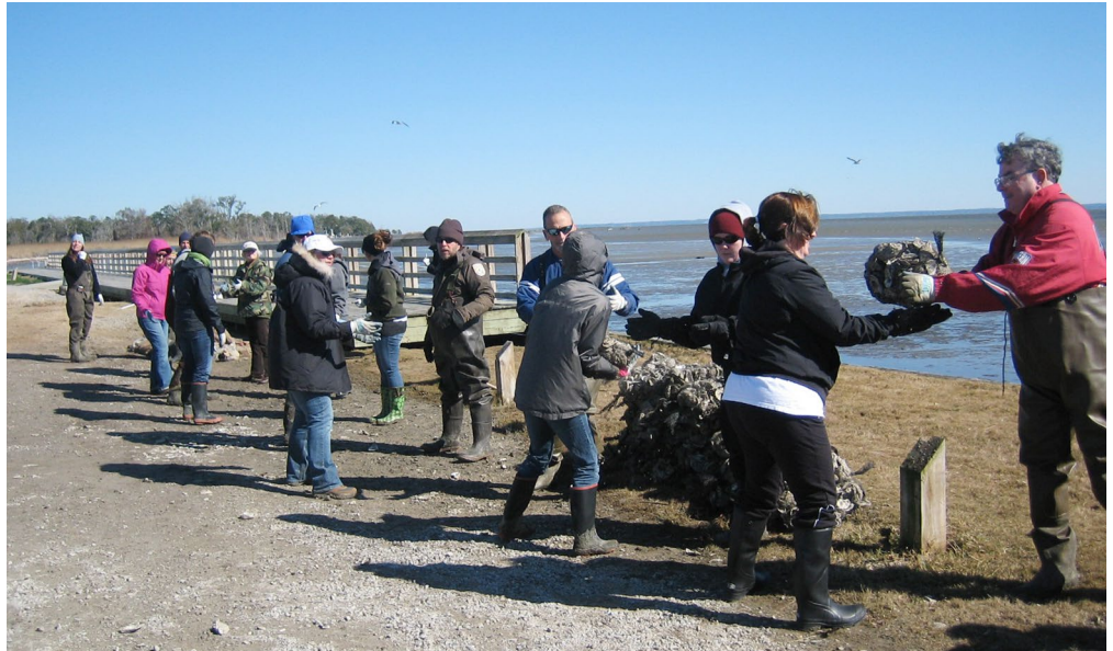
Partners installing an oyster reef in the City of Mobile's Helen Wood Park in south Alabama to provide important aquatic habitat, protect the shoreline from erosion, and act as a natural filter to improve water quality (USFWS).
