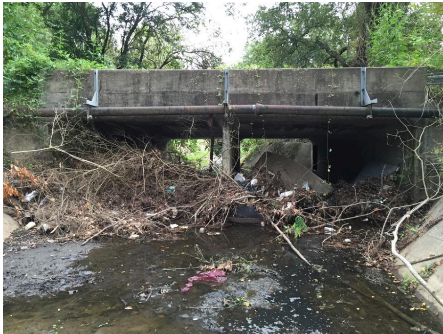
Figure 6. The channel is clogged by debris at the site 5
