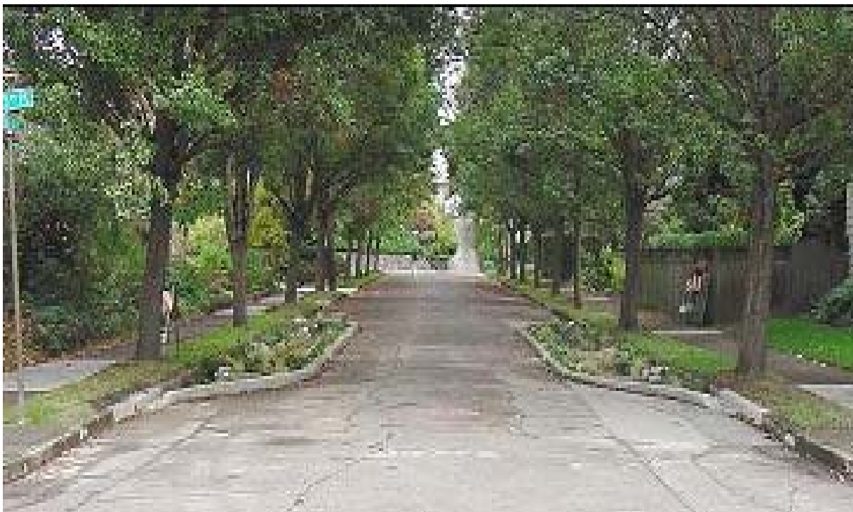
Figure 4-2 Example of Curb Extension (City of Portland – Bureau of Environmental Services, 2012)
