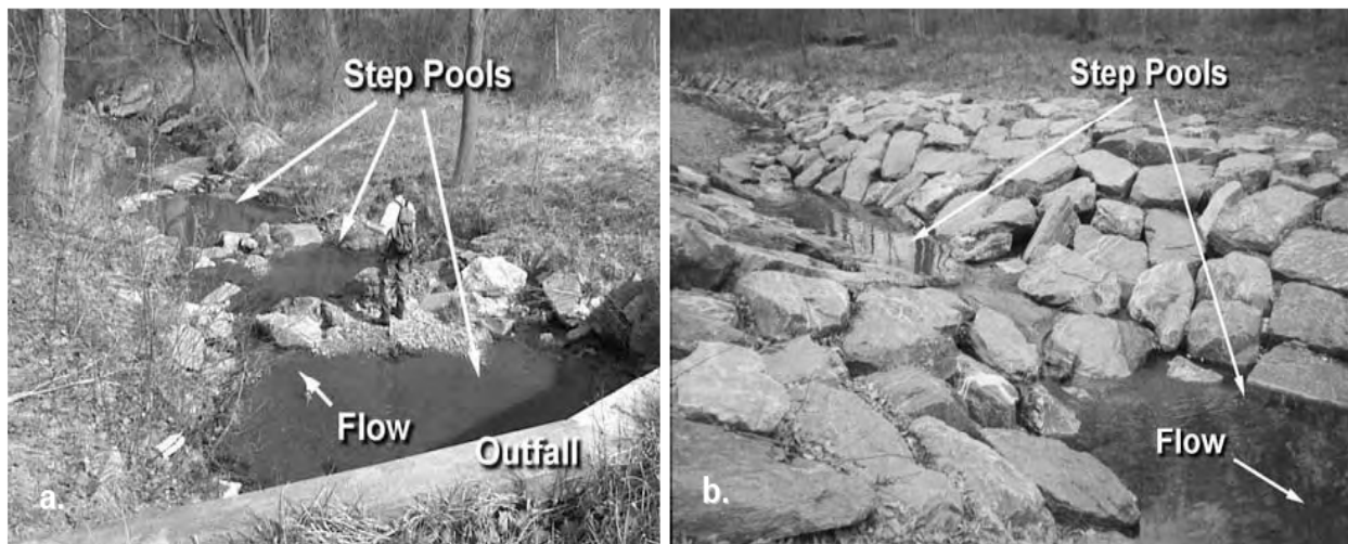
Figure 4-14 Step Pool Stream Restoration (CWP, 2004)
