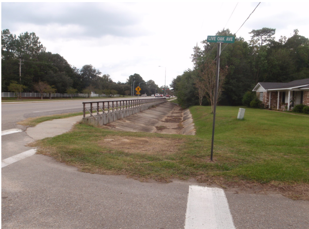
Figure 4-12 U.S. Highway 98/Greeno Road Ditches Lined with Concrete (JADE, 2011)
