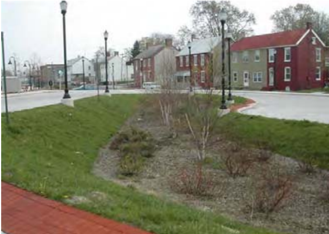
Figure 4-5 Example of Bioretention Pond (CWP, 2007)
