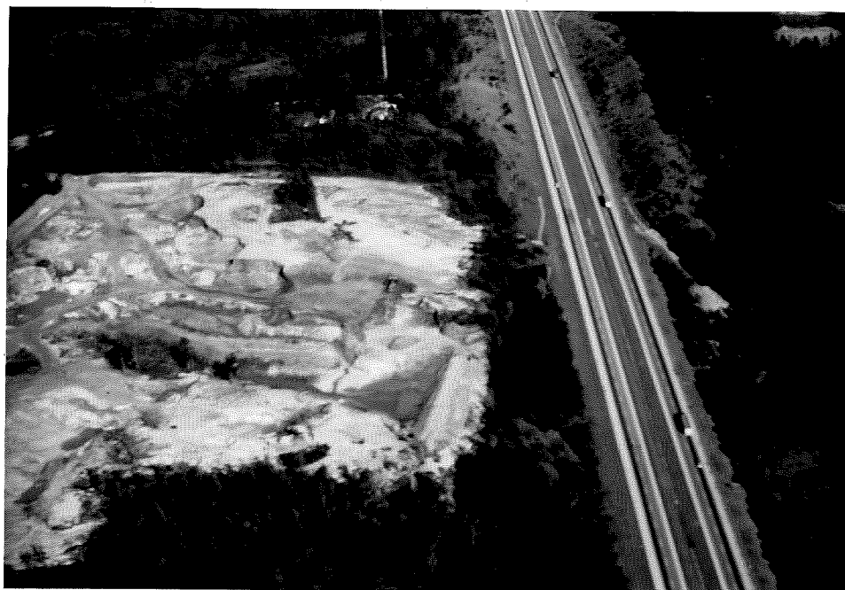
Fig. 9.--Sand pit in D'Olive Bay watershed located north of Interstate 10, operated by the Malbis Corporation (John Carlton photo, 1979).
