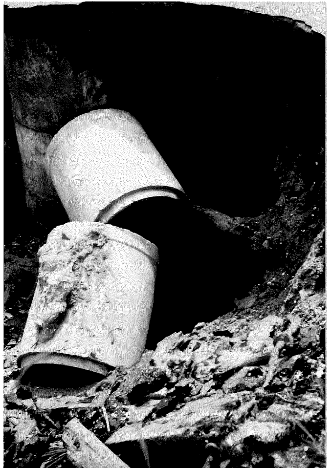
Fig. 17.--View showing broken culvert and undercutting of street (Lake Forest Estates, 1980).
