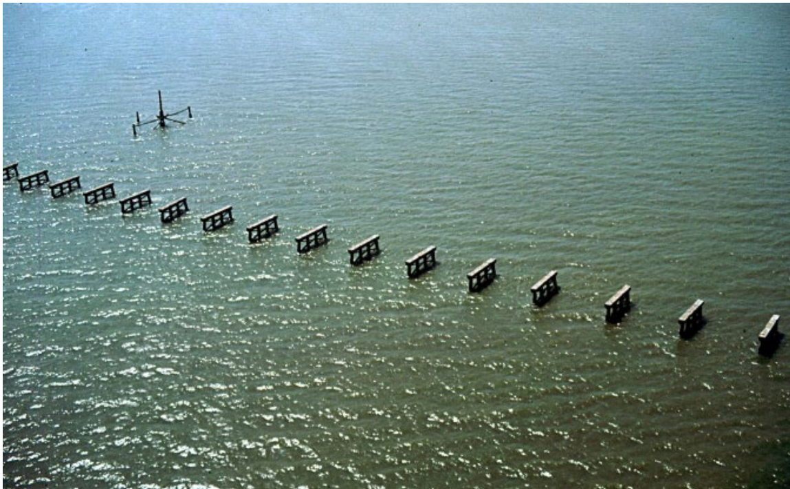
FIGURE 5-9 Photo of the Remains of the Dauphin Island Bridge after Hurricane Frederic
