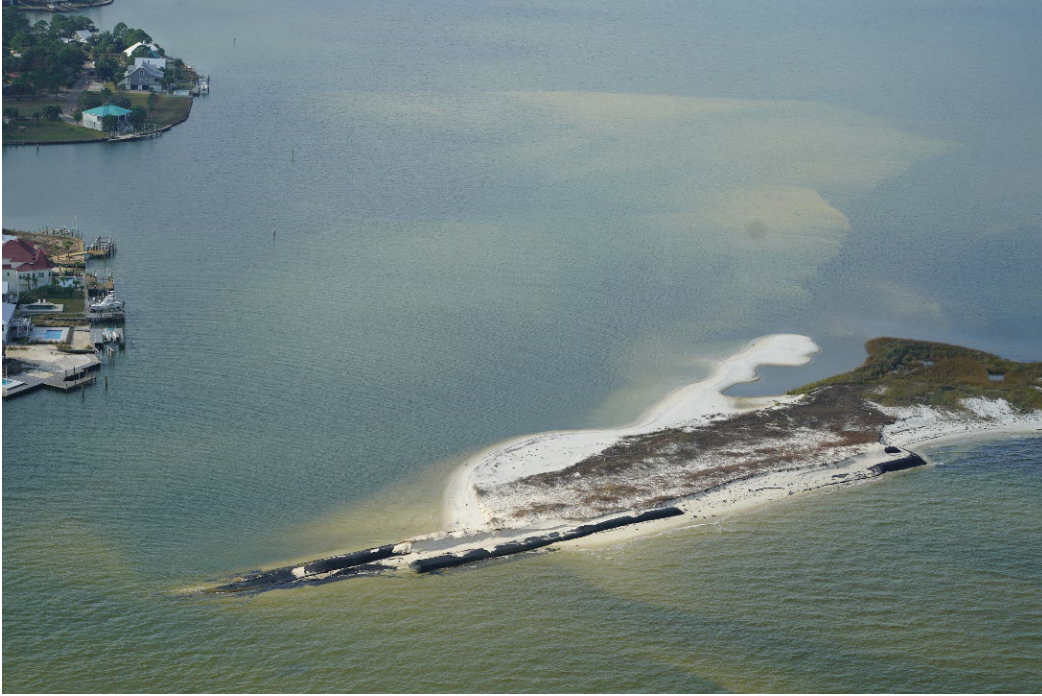
FIGURE 4-41 Shoreline Stabilization at Little Dauphin Island
