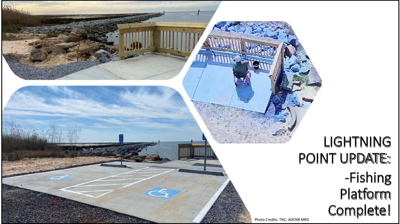
Funded through GOMESA the fishing platform is complete. Cost increases limited options, but a nice option was still constructed. Wheelchair accessible.
