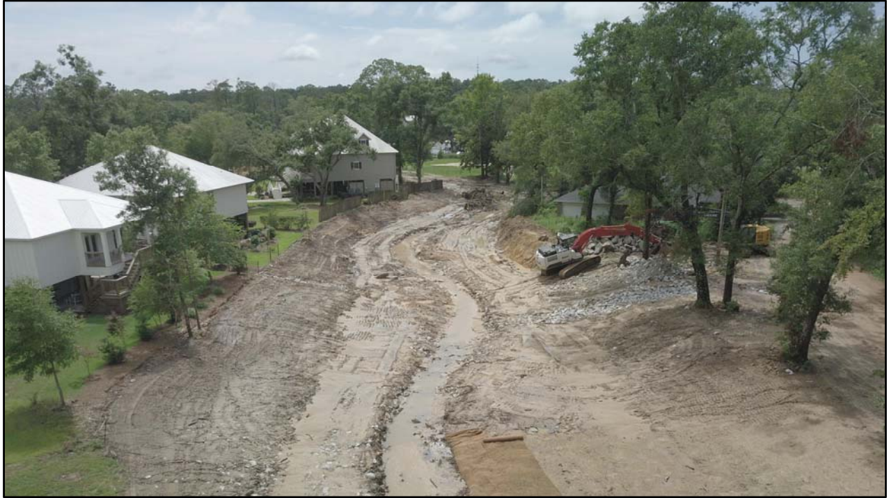
Photo of different phases of project construction.
