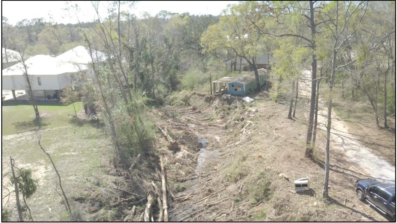
Photo of different phases of project construction.
