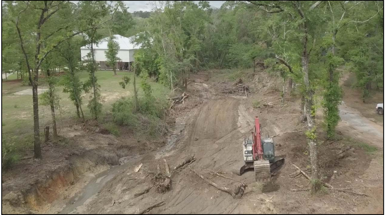
Photo of different phases of project construction.
