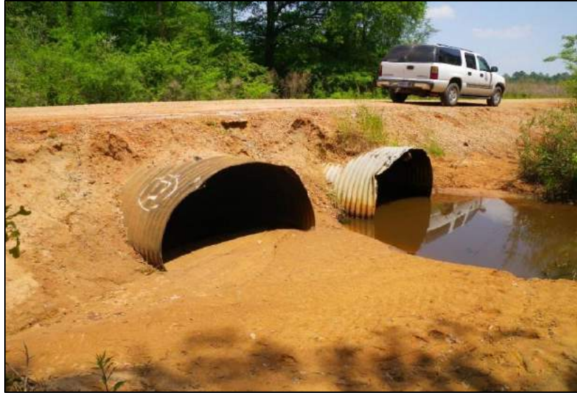
Figure 6.15 Unpaved road-stream crossing sedimentation
