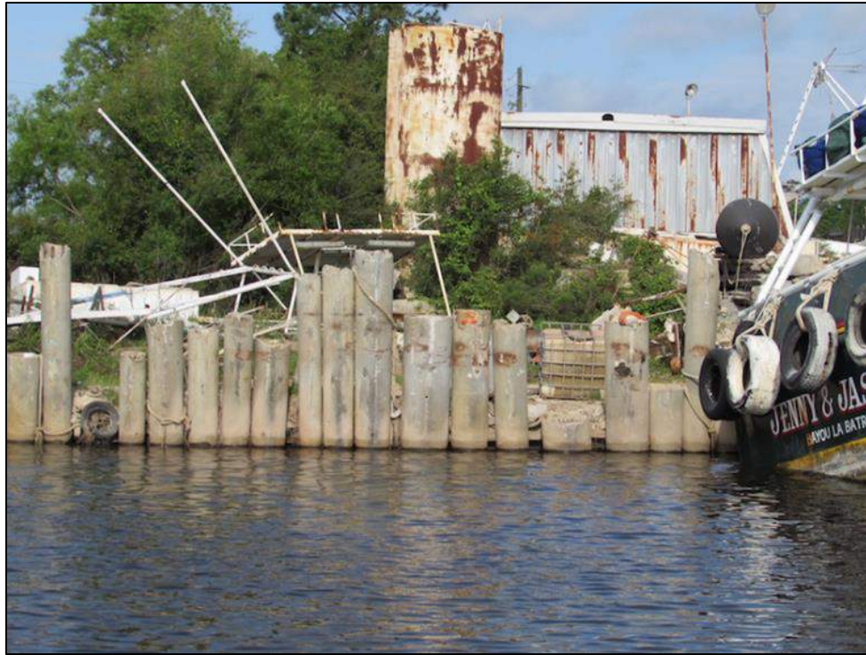
Figure 3.28 Typical example of failing or failed armored shoreline with upland erosion (Photo Credit Bret Webb)
