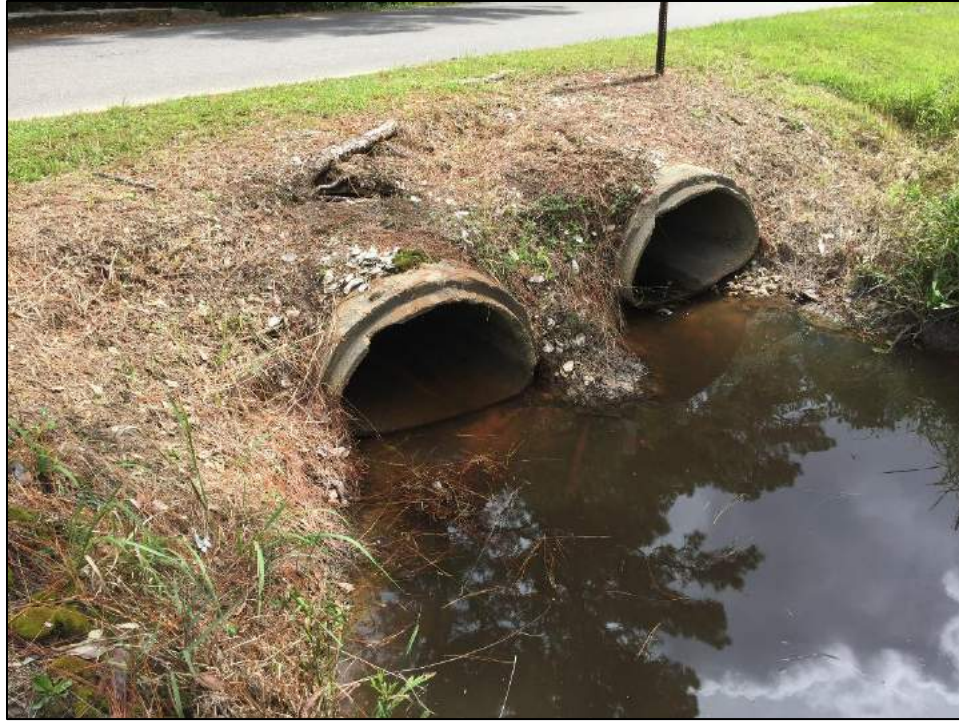
Figure 6.31 (1) Channel culvert crossing
