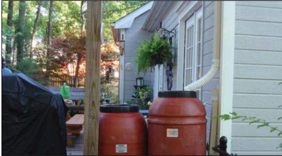
Figure 6.8 Example of rain barrel harvesting residential rainwater
