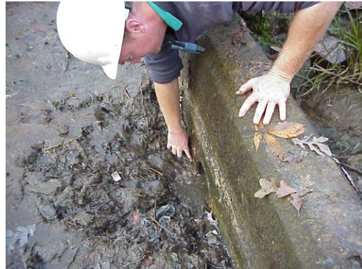
Figure M2.3: After clog is removed.
