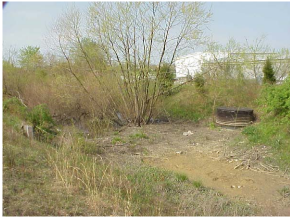
Figure 1.10: Sediment accumulation in a dry pond
