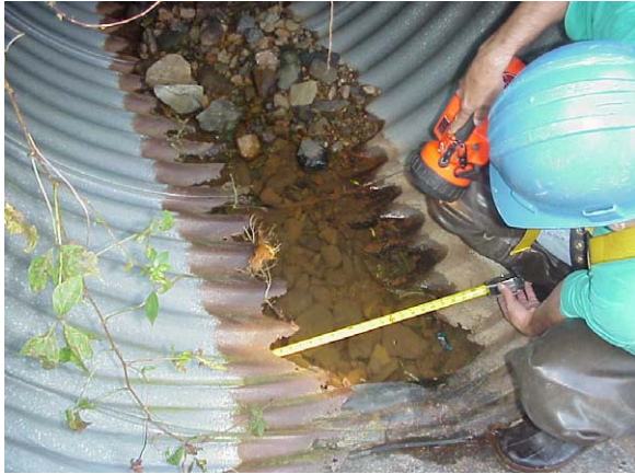
Figure 1.4: Pipe invert abrasion
