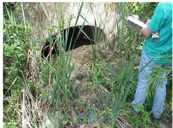
Figure M4.2: Excessive vegetation near an outfall.
