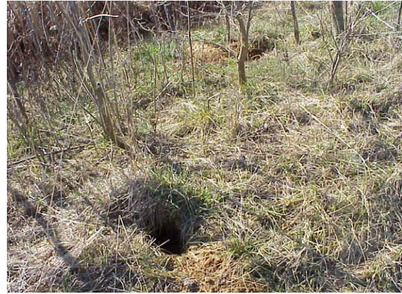
Figure 1.17: Animal burrow in pond embankment.
