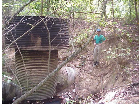
Figure 1.5: Severe erosion around riser and barrel
