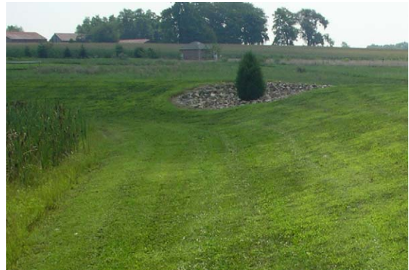
Figure M4.5: Unwanted vegetation - tree on embankment.
