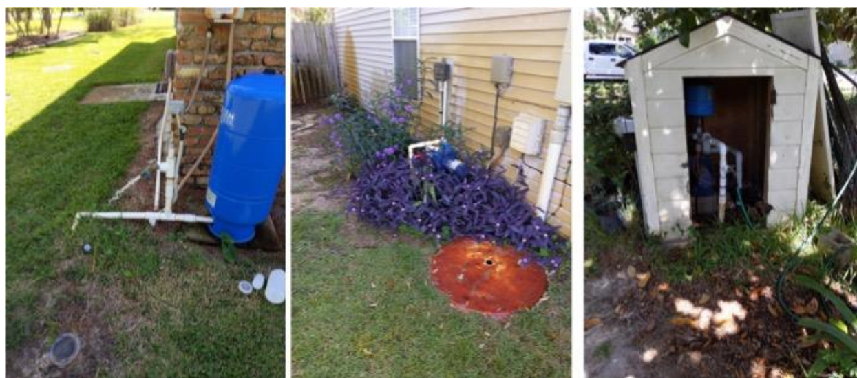
Figure 7 – Typical irrigation well infrastructure. All home owners reported using the same drilling service (Alm’s Pump Service Inc.), and drilling records posted online suggest installation depths within the shallow, surficial aquifer for all but one well. Water samples were collected from the well-head spigot following purging.
