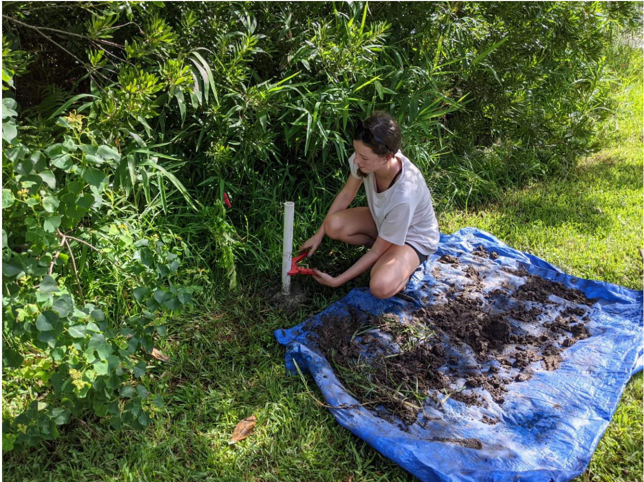
Figure 6 – USA researchers trims the top casing of a freshly installed well to final height. The sanitary seal can be seen on the ground surrounding the casing. Fresh auger cuttings are preserved on the tarp.
