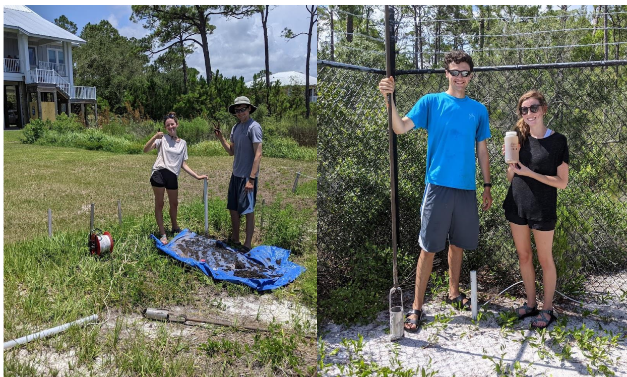
Figure 5 – USA researchers stand next to newly installed monitoring wells. The hand auger can be seen in the foreground of the left picture and being held by one of researchers in the right picture. Casings were trimmed to approximately 15-20 cm above ground surface.
