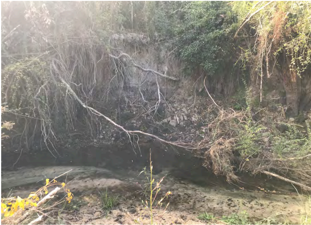
Photo B3. RSA1, downstream portion of the survey transect.
